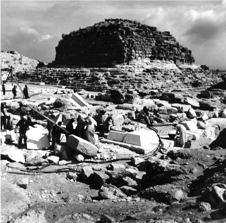
Fig. 17. West side of the satellite pyramid, looking northeast.
